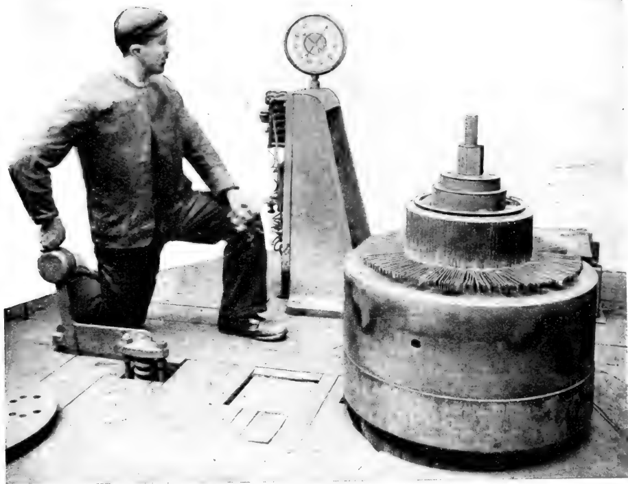
FIG. 132.—200-ton Press for squeezing Commutators. Vickers, Sons & Maxim.
